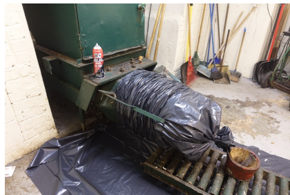
Garbage disposal room
